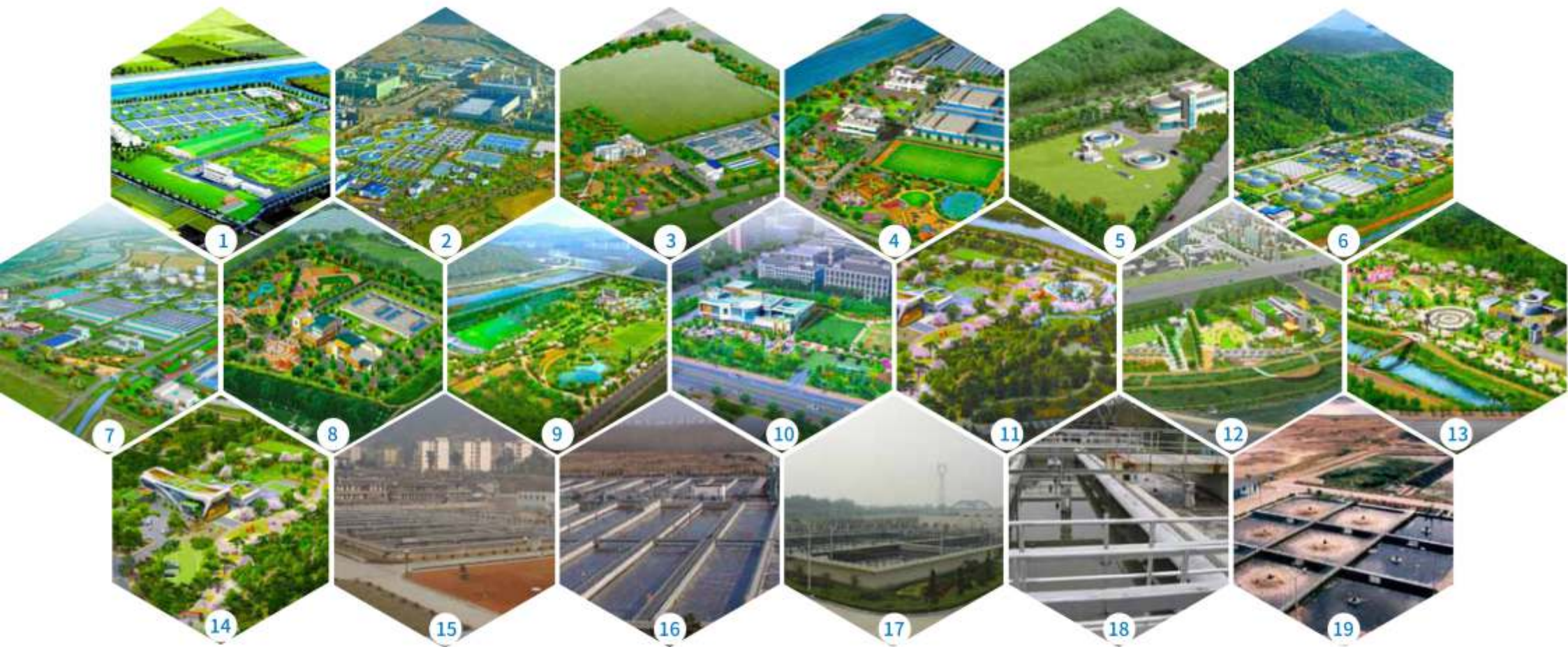
1. Suwon Phase-1 WWTP (220,000m 3 /d)
