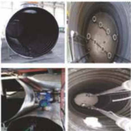
Reactor equip. installation (Diuser/pump/pump/discharge device)
